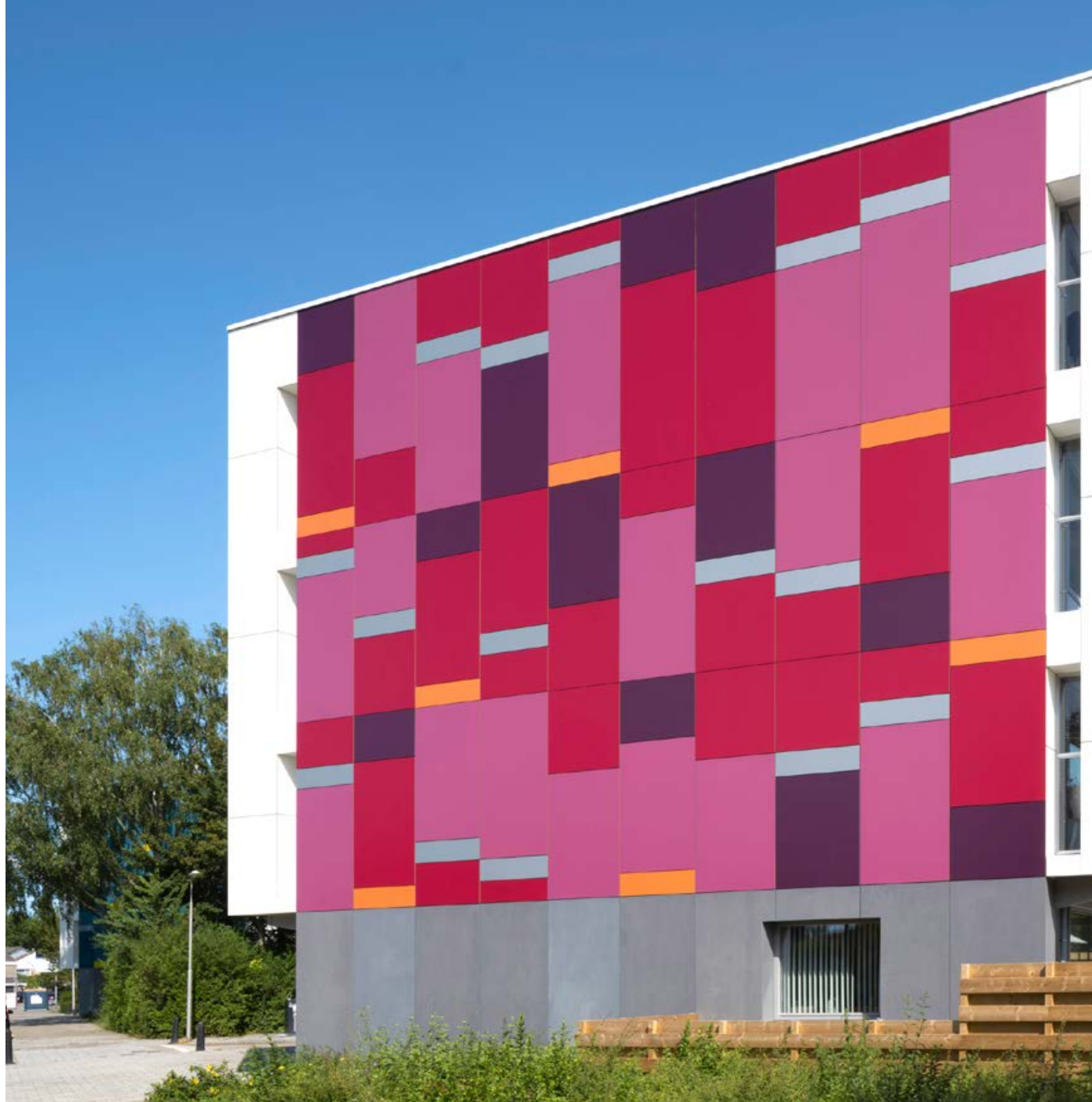
Project: Renovated flats, Emmeloord, The Netherlands
