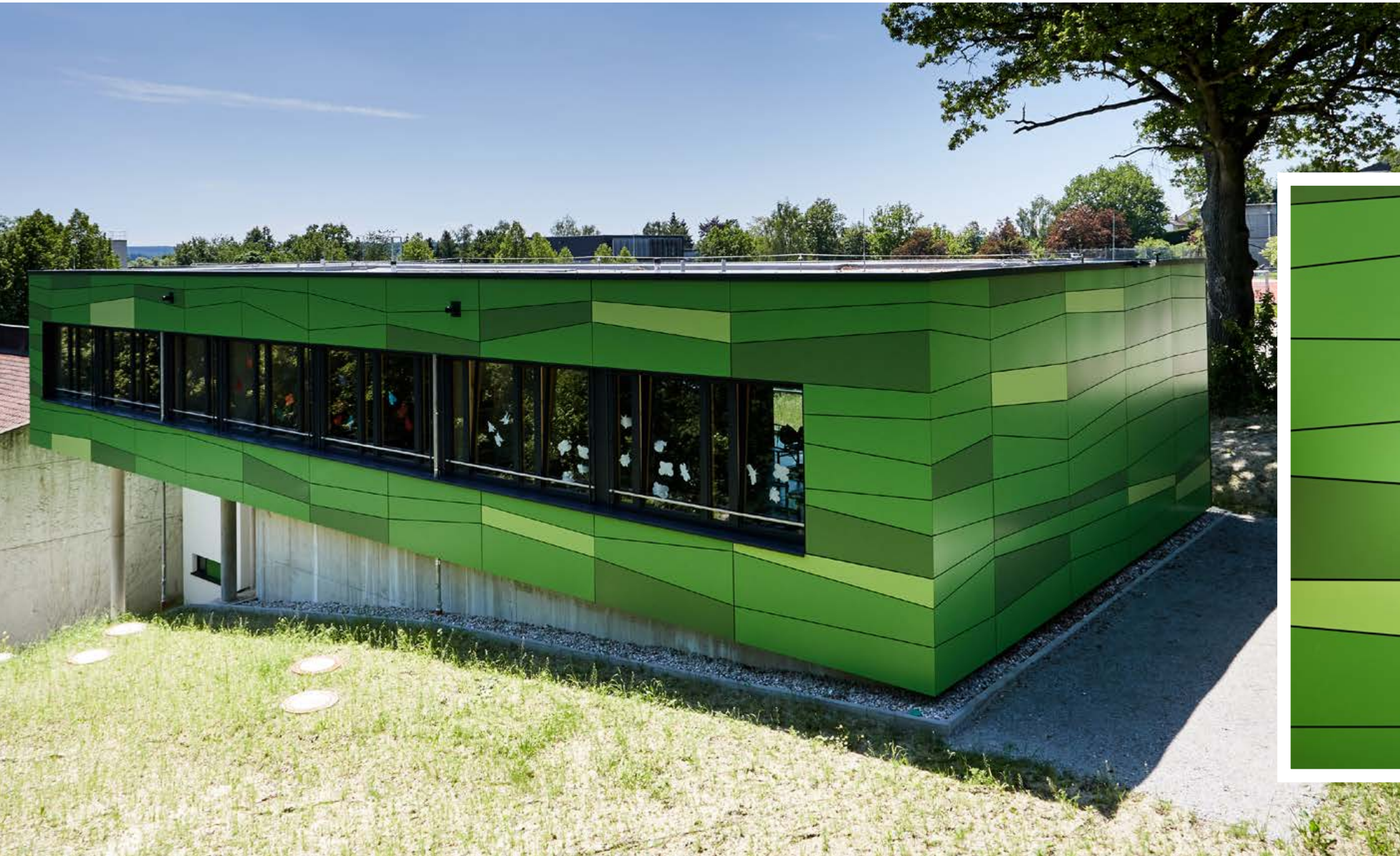
Project: Betty-Greif-School, Pfarrkirchen, Germany
